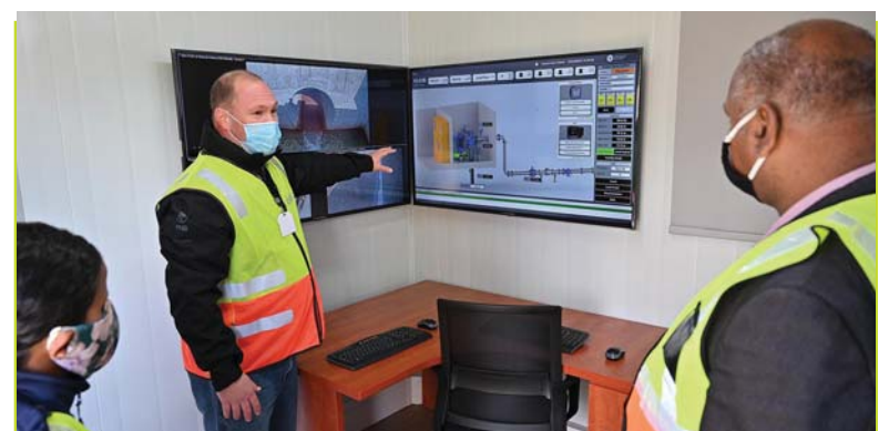
Well, well, well: The new Steenbras groundwater wellfield is controlled remotely.
